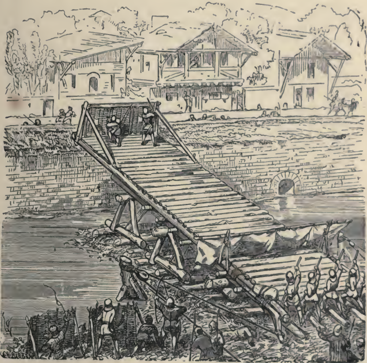
FIG. 26.—THE ATTACK—THE MOVABLE BRIDGE INTENDED FOR CROSSING THE SMALL ARM OF THE RIVER OF ARONIA.
